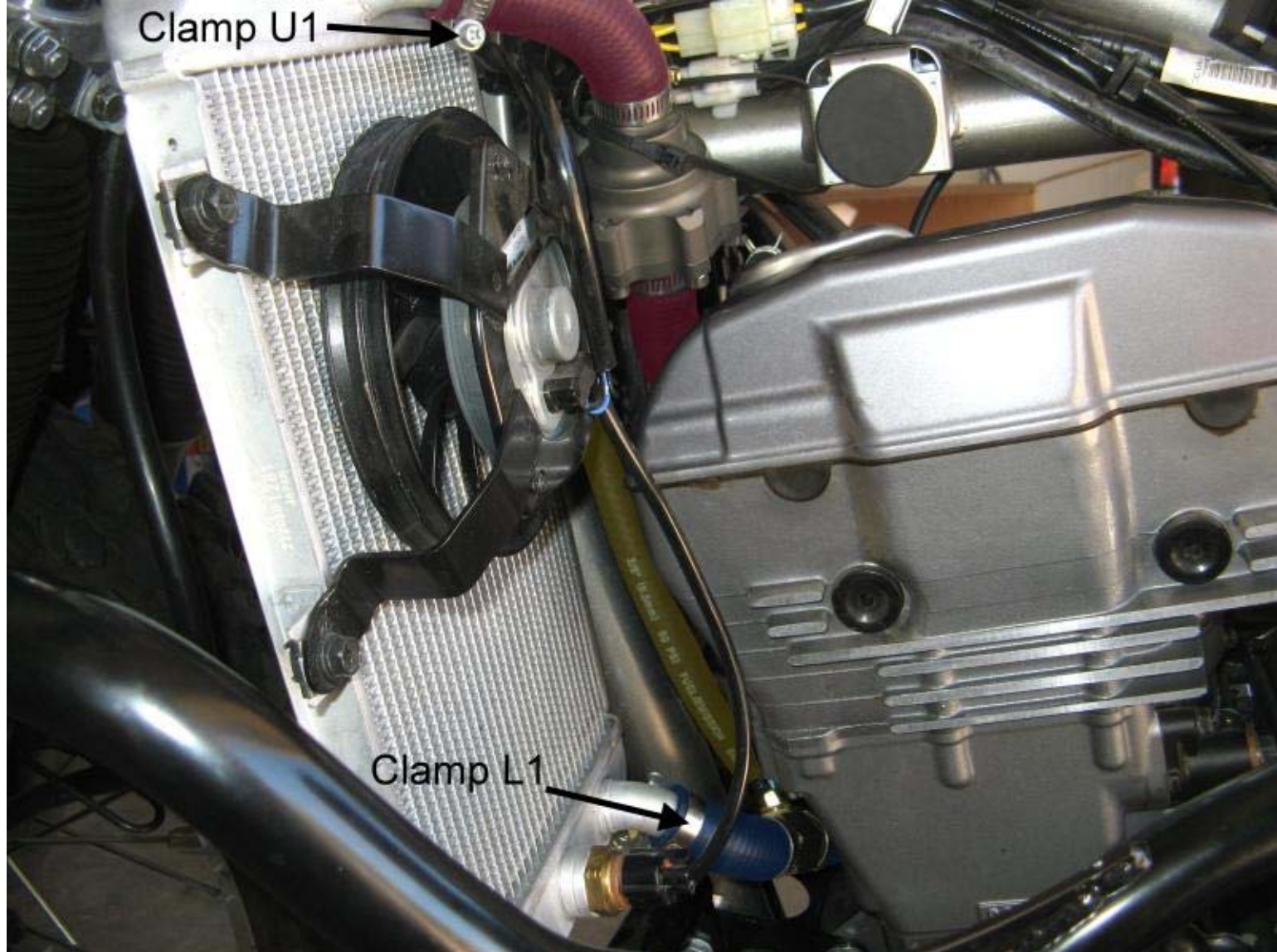
Figure 4: Completed Installation. Hoses have been color coded to help in identification; red/purple is upper radiator hose, blue is lower radiator hose, gold is new bypass hose.
